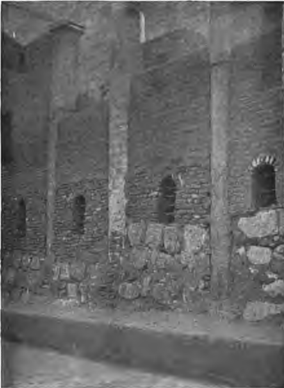
FIG. 143.—The White Monastery: Wall-in columns of nave. (Photo. by J. G. M.)
